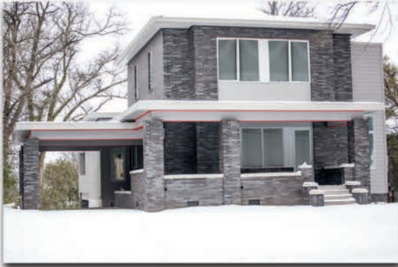
400 RHETT STREET, GREENVILLE, SC before clean up of Utility poles and lines
